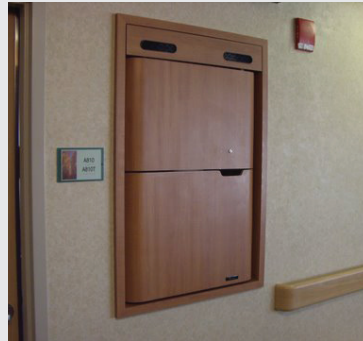
5. Protrudes no further than a chair rail.
